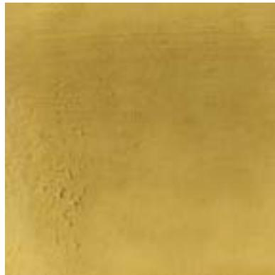
Example of 'mud cracking' when substrate hasn't been correctly 'damped down' or limewash dilution rates are not correctly observed
