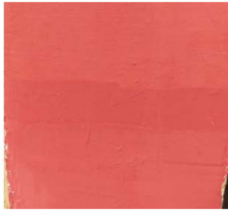
Example of visible bands from leaving straight wet edges, feather out limewash to help avoid banding
