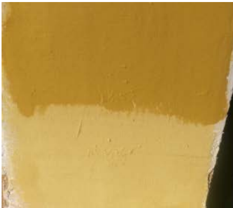
Example of a straight wet edge, do not leave a straight wet edge as 'banding' can occur'
