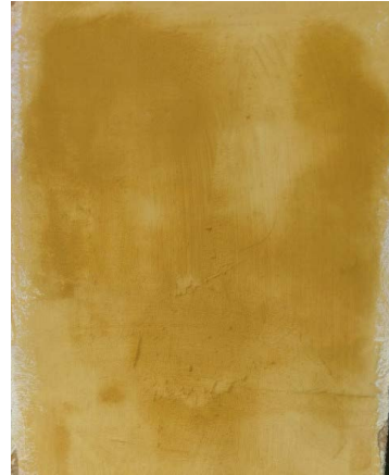
Limewash During Drying
